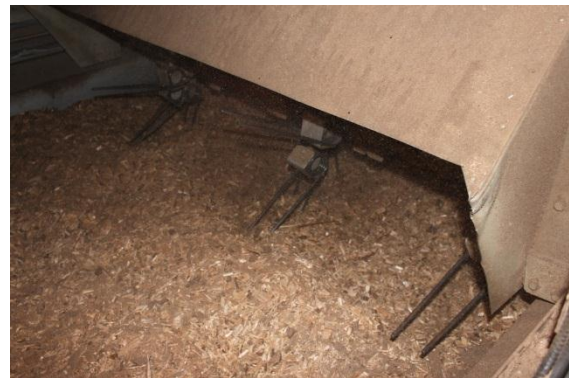
Figure 43: Paddles of a feed-and-turn drier mixing woodchips (Source: Rutz)
