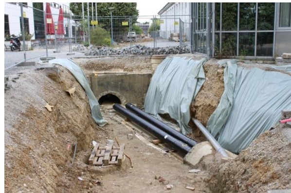
Figure 19: Construction of a district heating system in Germany (Source: Rutz)
