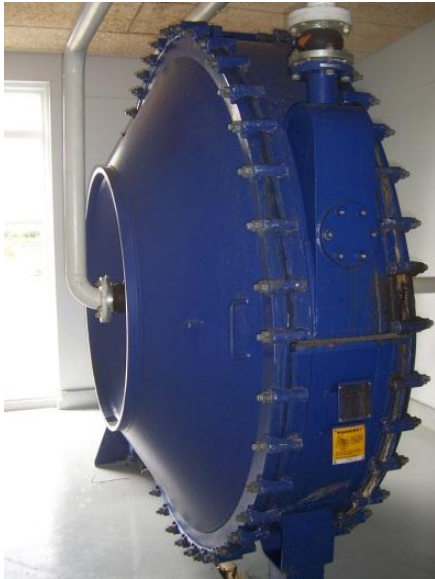
Figure 20: Spiral heat exchanger in Denmark (Source: Rutz)
