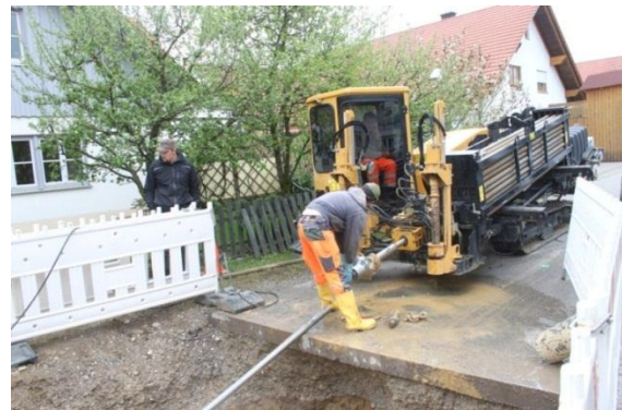
Figure 13: Directional drilling machine (Source: Rutz)
