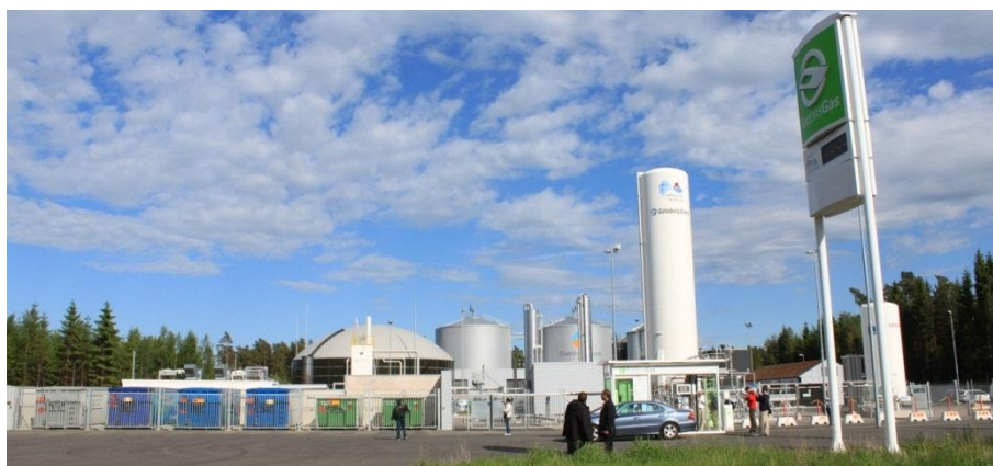
Figure 69: Biogas plant of Swedish Biogas International producing LBG in Lidköping, Sweden (Source: Rutz)
