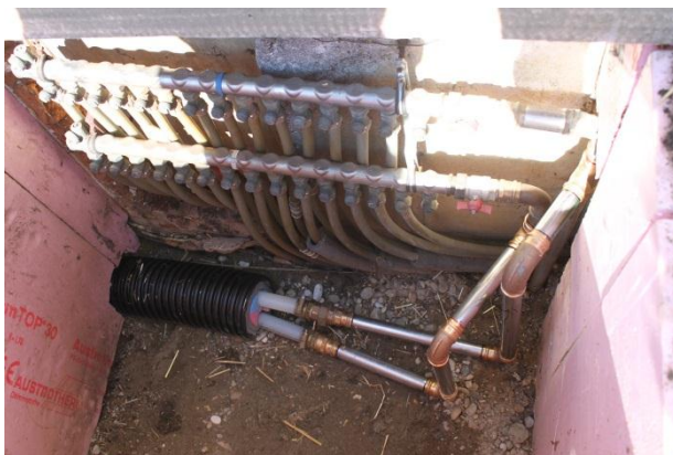
Figure 16: Installed PE twin-pipe for digester-heating (Source: Rutz)
