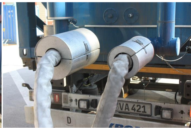
Figure 33: Insulated docking station of a heat storage container (Augsburg, Germany) (Source: Rutz)
