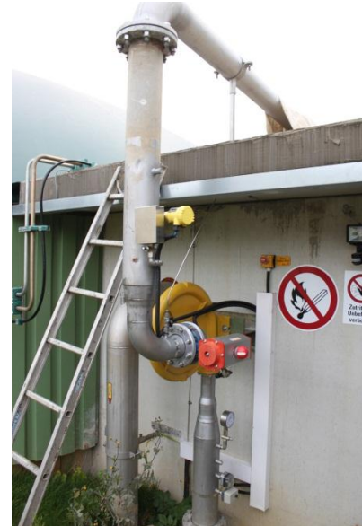
Figure 64: Start of a biogas pipeline (including the ventilator) to a satellite CHP unit in Germany (Source: Rutz)
