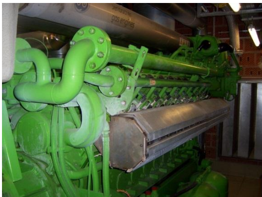
Figure 9: Gas-Otto engine in a biogas plant in Germany (Source: Rutz)
